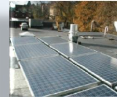
PV panels under test
