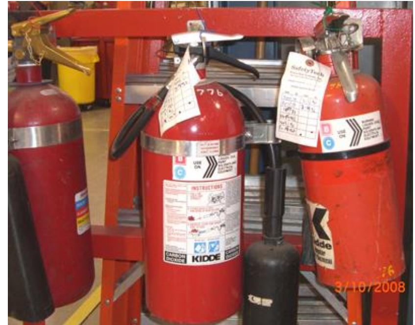
Fire Extinguishers (20# Size shown)
