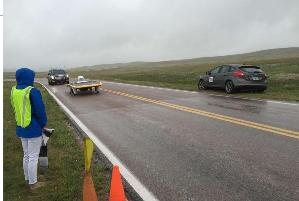
Good vehicle placement but flagger should be in front of LV and don't use road side doors
